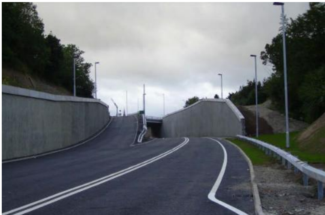
Fig 8 – Insertion of single-track railway into Omagh Throughpass (Dublin Road example) can be accomplished by bringing the line in along the landstrip to the right of the photo, and behind the retaining wall extending out from the road bridge, with a new road bridge across the line to the right (out of sight). Alternatively, the retaining wall could be moved to the right and the visible road bridge extended. These are just some engineering possibilities that can be considered at the design stage.
